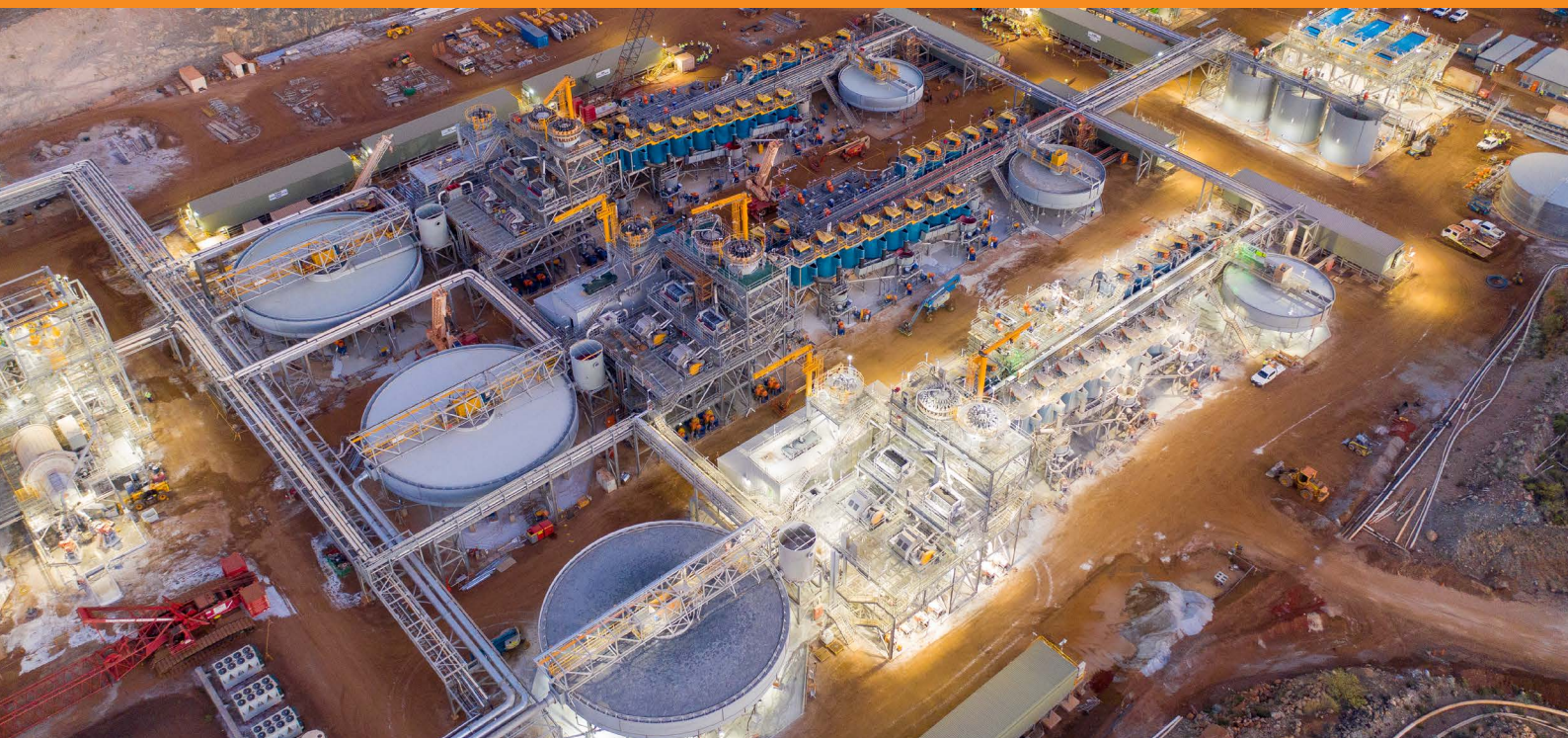
Cover and above photo: The crushing plant and beneficiation plant at Mineral Resources' Wodgina Minesite
