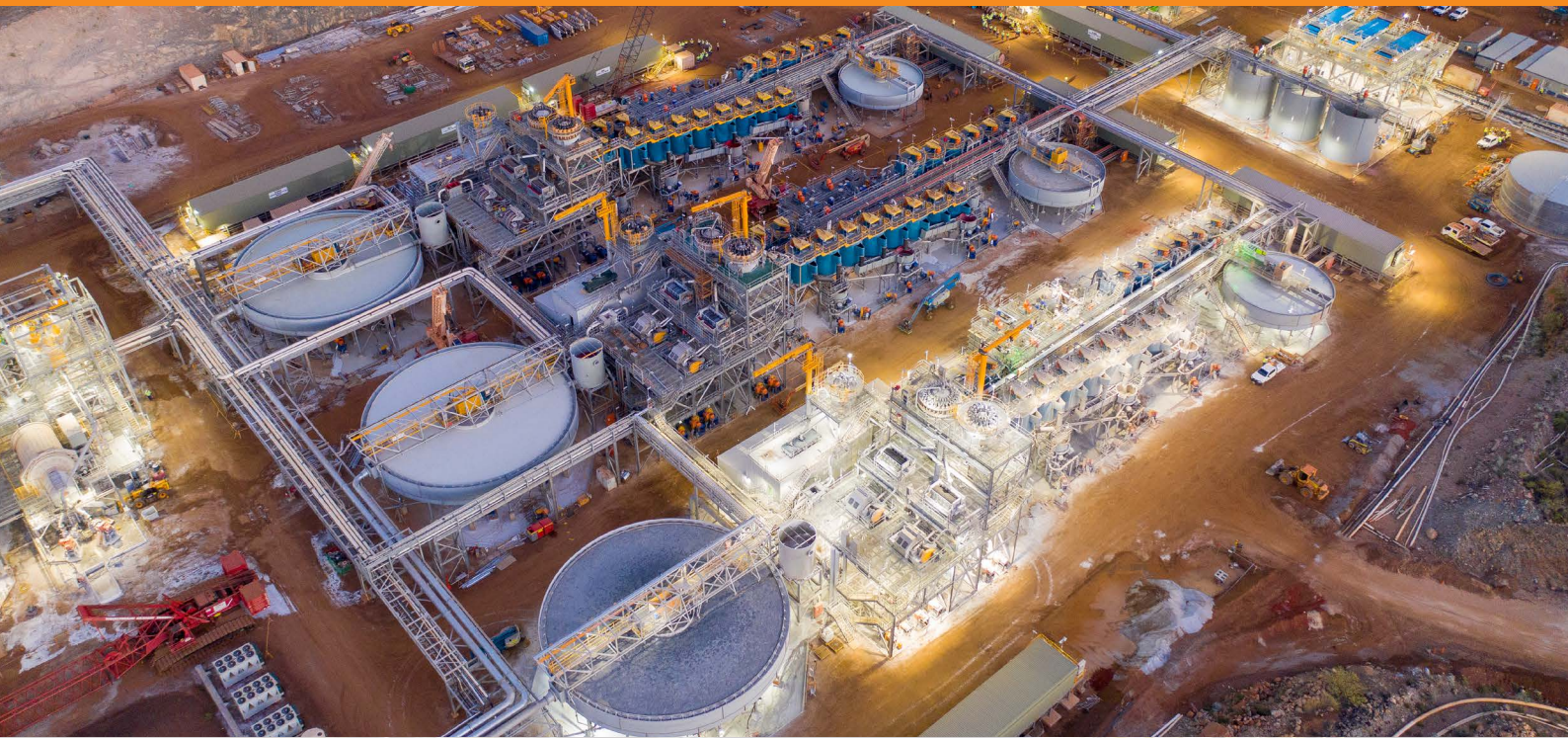
Cover and above photo: The crushing plant and beneficiation plant at Mineral Resources' Wodgina Minesite
